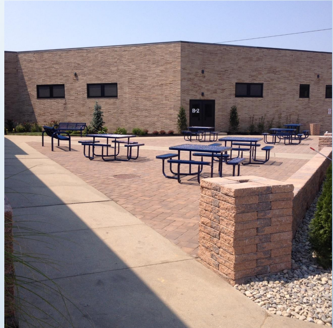
Highland Paver Patio Installed In-House
